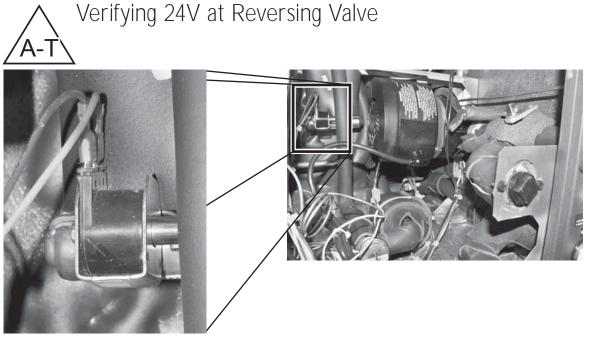
Verify 24V at reversing valve when calling for cooling
