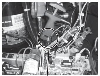
3) Clamp on the meter close to the sensor location
