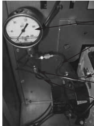
FIGURE 18 OIL PRESSURE TESTING ASSEMBLY INSTALLED
