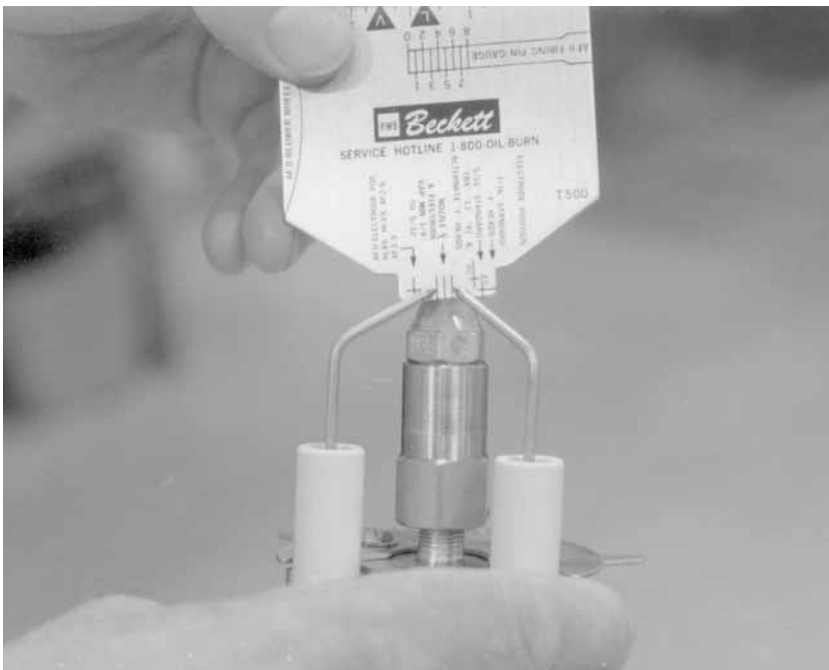
FIGURE 20 ELECTRODE ADJUSTMENT
